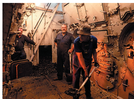
The boiler room 'stokers'
